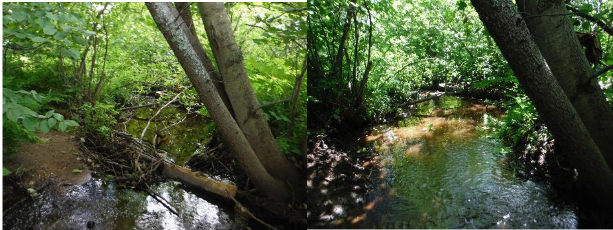
FIGURE 5. BEFORE AND AFTER OF A DEBRIS BLOCKAGE REMOVAL DOWNSTREAM FROM A CULVERT ON MCLEAN BROOK.
