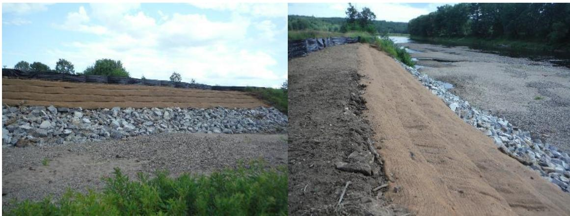
**FIGURE 8. IMMEDIATELY AFTER COMPLETING THE EROSION CONTROL BLANKETS AND BEFORE ANY PLANTING WORK WAS DONE. THE SEDIMENT FENCE WAS MOVED TO THE TOP TO PREVENT PEOPLE FROM TAMPERING WITH THE SITE.**
