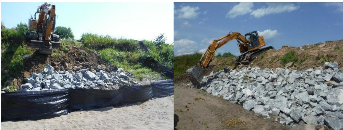
**FIGURE 6. LEFT: THE EXCAVATOR PLACING THE FIRST SECTION OF R250 MIXED RIP-RAP IN THE TRENCH AT THE TOE OF THE SLOPE. THE SEDIMENT FENCE IS PROTECTING THE WATERCOURSE FROM SEDIMENTATION. RIGHT: THE EXCAVATOR PLACING THE FINAL SECTION OF R250 RIP-RAP AT THE TOE OF THE SLOPE.**
