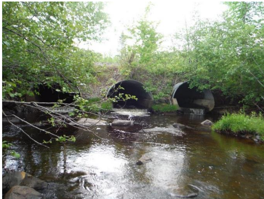
Figure 6. This triple culvert on Manzer Brook is a barrier to fish as all three culverts have outflow drops of between 38 and 62 cm. We are working on a remediation option to reinstate fish passage.
