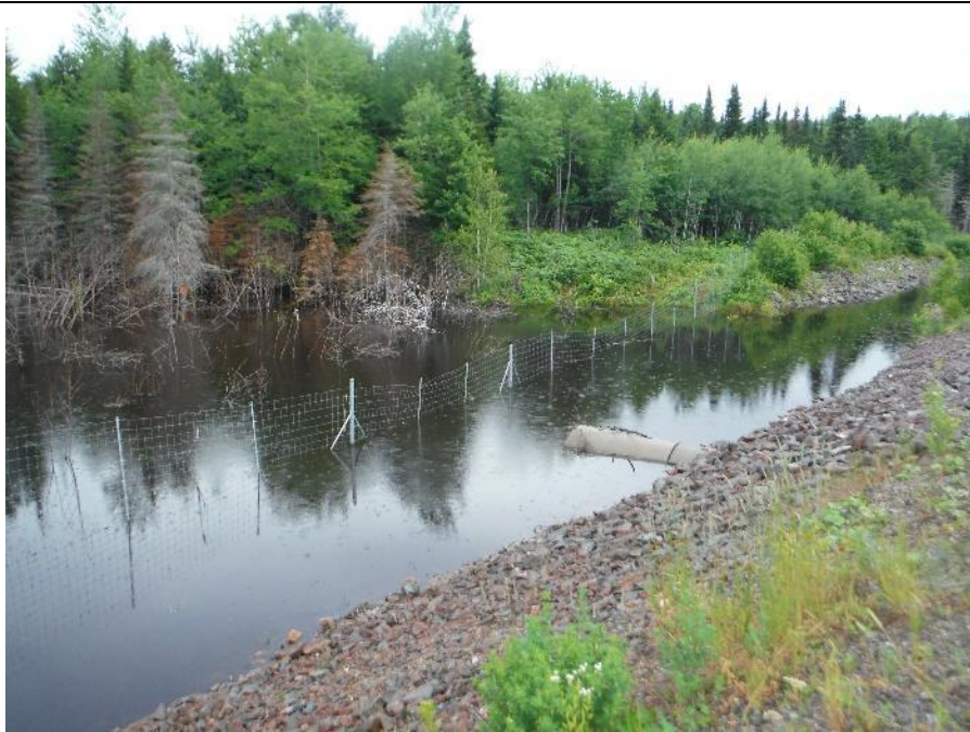
Figure 3. Beavers have flooded the upstream portion of this small stream by blocking the inlet of the culvert.
