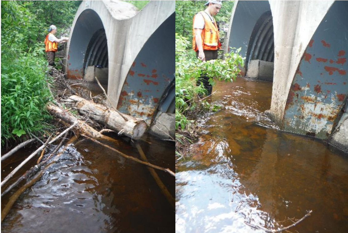
Figure 4. A debris blockage between culverts 2 and 3 at a culvert on Manzer Brook was removed, which improved the flow of water. Culvert 1 has a large tree inside of it that could not be removed with the equipment we had.
