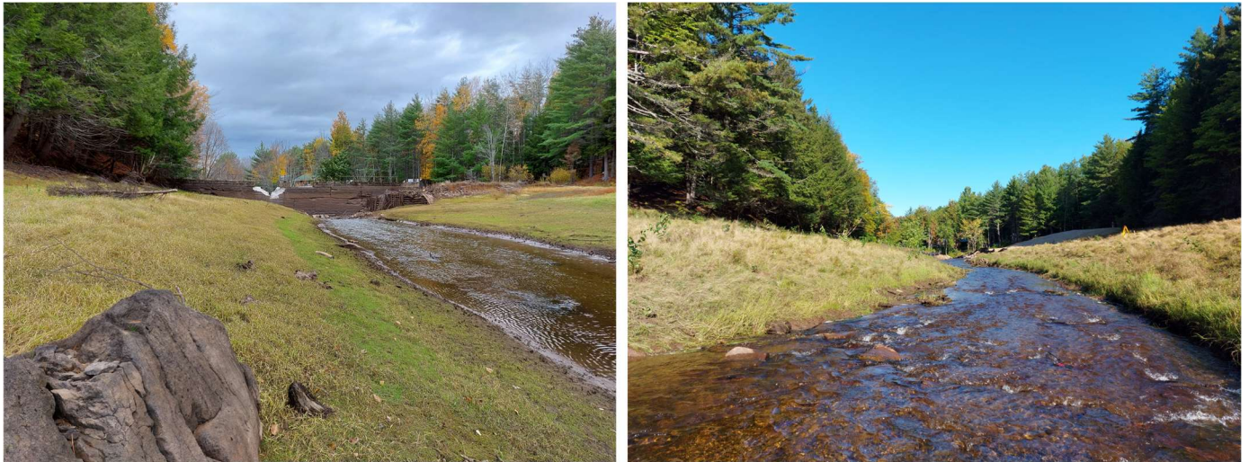
Figure 1. LEFT: Campbell Creek prior to removal in fall 2020, RIGHT: Campbell Creek post dam-removal and tree planting in fall 2021. As can be seen in the image on the right, the former stream channel, comprising gravel beds and bedrock has now been exposed and flushed of silt that had accumulated in the headpond.
