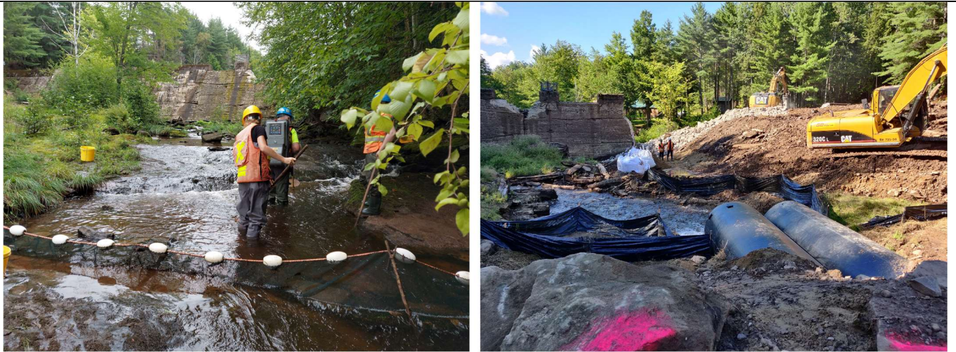
Figure 2. LEFT: Photo of one of several fish rescues conducted throughout the dam removal process. RIGHT: Dam removal, mid-construction. The creek channel was diverted several times during this process.
