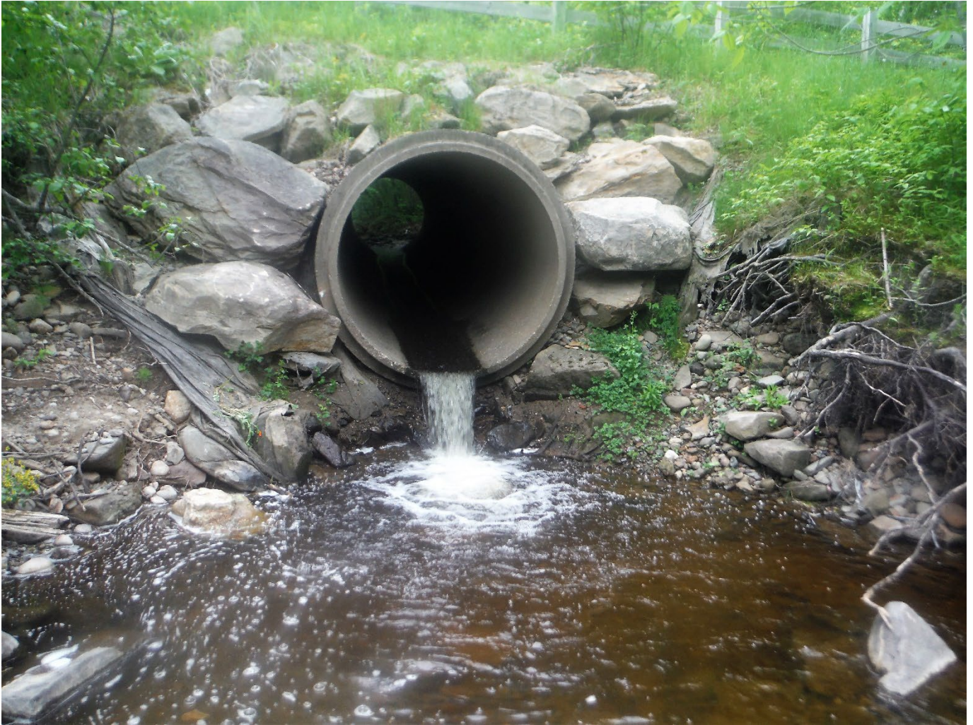
Figure 10. McConaghy Brook (MCC02) culvert outflow looking upstream. Picture taken in 2017.
