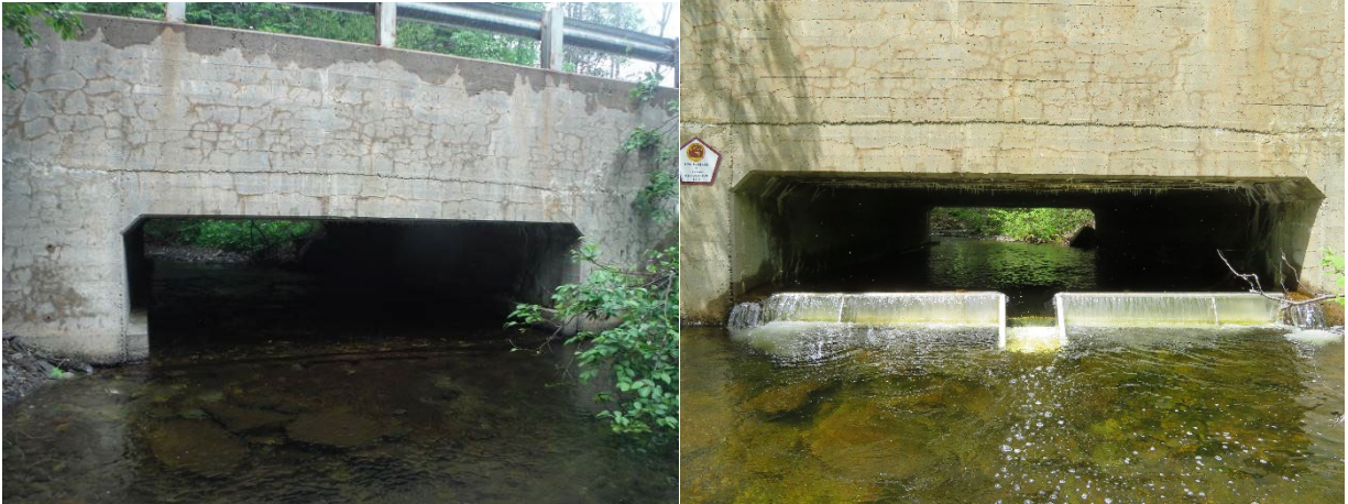
Figure 6. Before and after of the McGivney Brook fish passage project. Picture on the right was taken during a site check in 2023.
