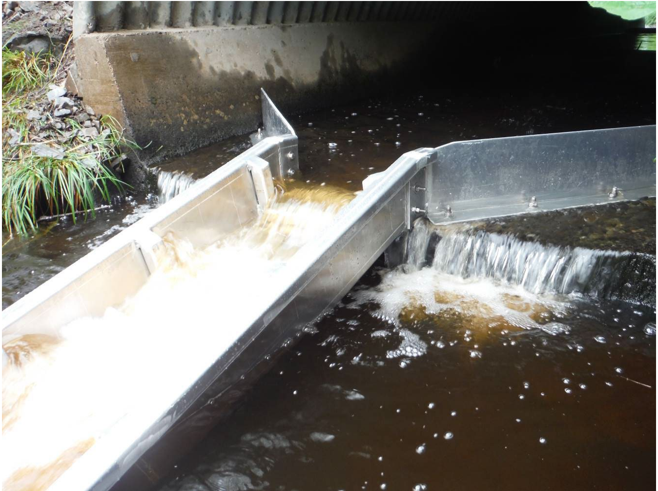
Figure 3. The Manzer brook fish ladder, installed in August 2018.
