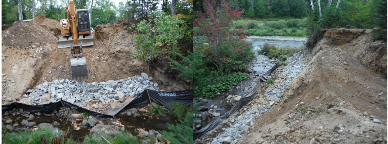
Figure 7. Step 3. R50 riprap was mixed with existing rocks and placed in a trench at the toe of the slope.
