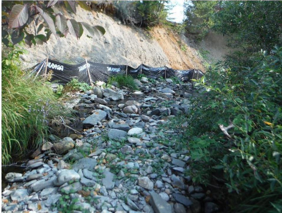
Figure 5. Step 1. A sediment fence was installed before work began.
