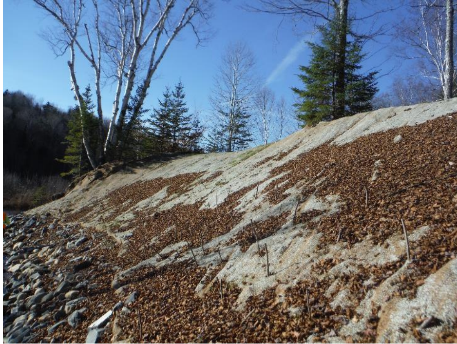
Figure 11. Tree seedlings were planted on top of the bank while willow stakes were planted in the lower half of the bank.
