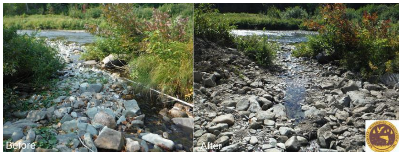
Figure 18. Looking downstream at the mouth of MacPherson Brook before (left) the rock weir was installed, a gravel island had built up and was channeling water to either side, which was causing more bank erosion. After (right) the installation of the sunken rock weir at low flow conditions.
