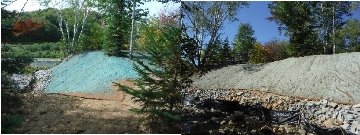
Figure 9. Step 5. The erosion control blankets were rolled up and hydroseeded. >200 willow stakes were planted in the lower half of the bank.
