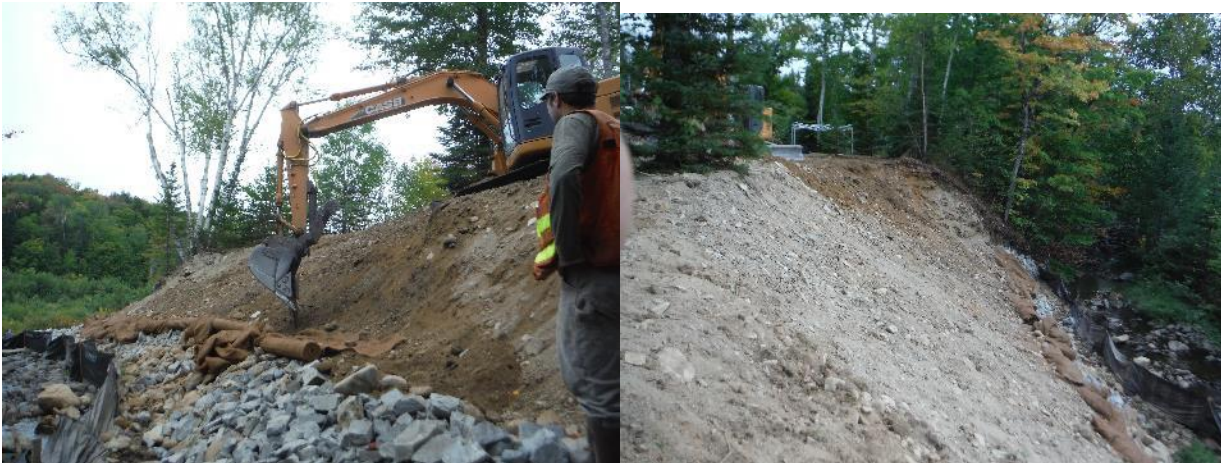
Figure 8. Step 4. The erosion control blankets were laid on top of the rock toe and dirt was place on the end on the blanket to hold it in place before the blankets were rolled up over the slope. Not shown is a layer of hay that was placed under the blankets.
