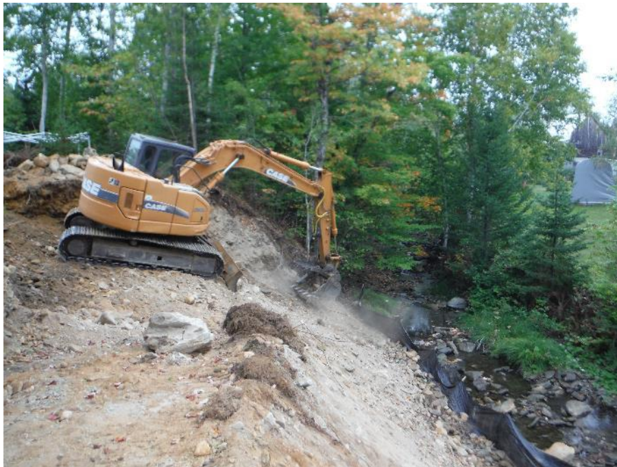
Figure 6. Step 2. We began reshaping the bank and digging the trench where the R50 would be placed.
