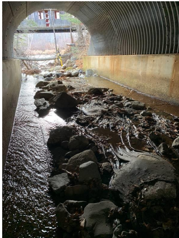
Figure 10. This pipe on Sands Brook on Giant's Glen road has experienced major deterioration of the substrate in the last few years. Though it has open bottom it appears as though this culvert is no longer passable to fish. Black sediment control fabric is shown exposed in the photo above.
