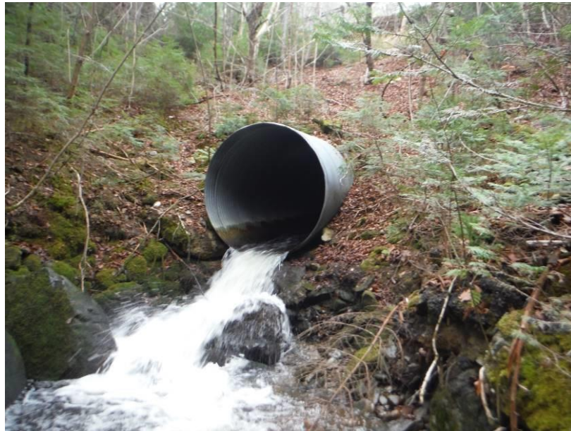
Figure 8. The Porter's Brook culvert on Nashwaak West road is a severe barrier to fish. The pool at the mouth of this brook is an important salmon holding pool that DFO closes annually on June 15. Nashwaak West Road has been closed for many years and will not reopen. If this culvert blows out in a storm, the brook, the pool at the mouth of the brook, and downstream habitat in the Nashwaak River will be irreversibly damaged.
