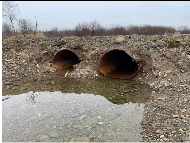
Figure 9. This pipe on McLean Flats Roads is in very poor shape and fills with gravels annually during the freshet. These pipes need to be replaced. Local residents described many fish including Atlantic salmon using this stream in previous years.
