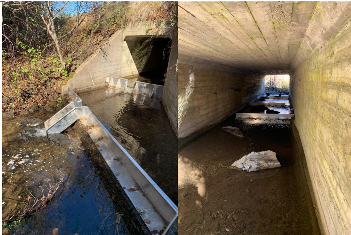
Figure 4. Details of the East Ryan Brook fish passage project showing the chute and first two baffles (left) and the upper three partial baffles (right) as well as the large rocks placed to provide microhabitat in the pipe.
