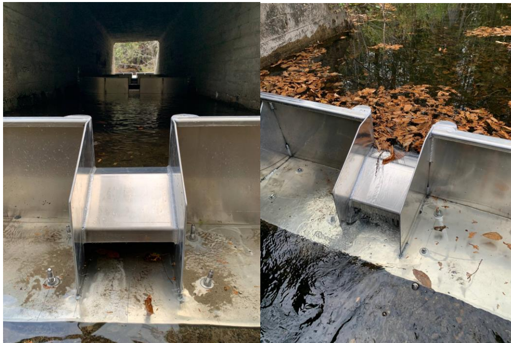
Figure 7. A close up shot showing the weirs installed for the Limekiln Brook fish passage project. The weirs were not fully installed at this point so water was just starting to flow over the chute.
