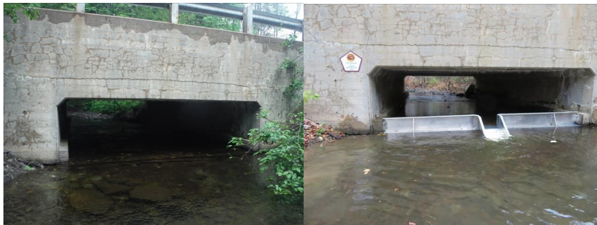
Figure 5. Before and after of the McGivney Brook fish passage project
